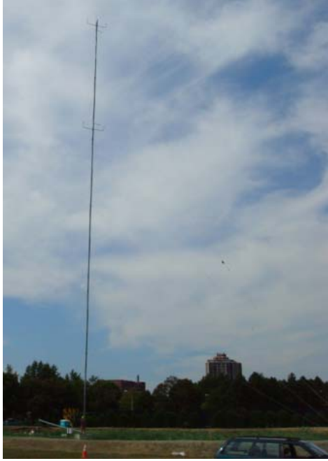
The new MET tower that will determine whether wind turbines are an option for generating energy at Harvard.
