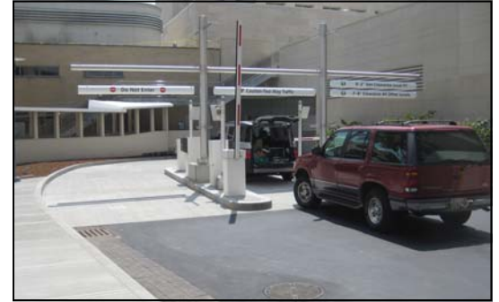
The entrance to the new Everett Street Garage
