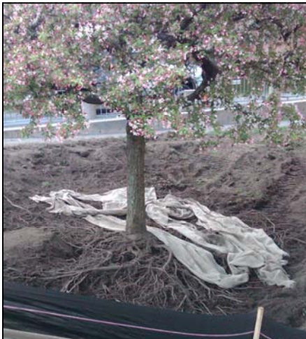
Using an air-spade, a wide swath of soil is removed, exposing the vast root system which is then carefully removed.
